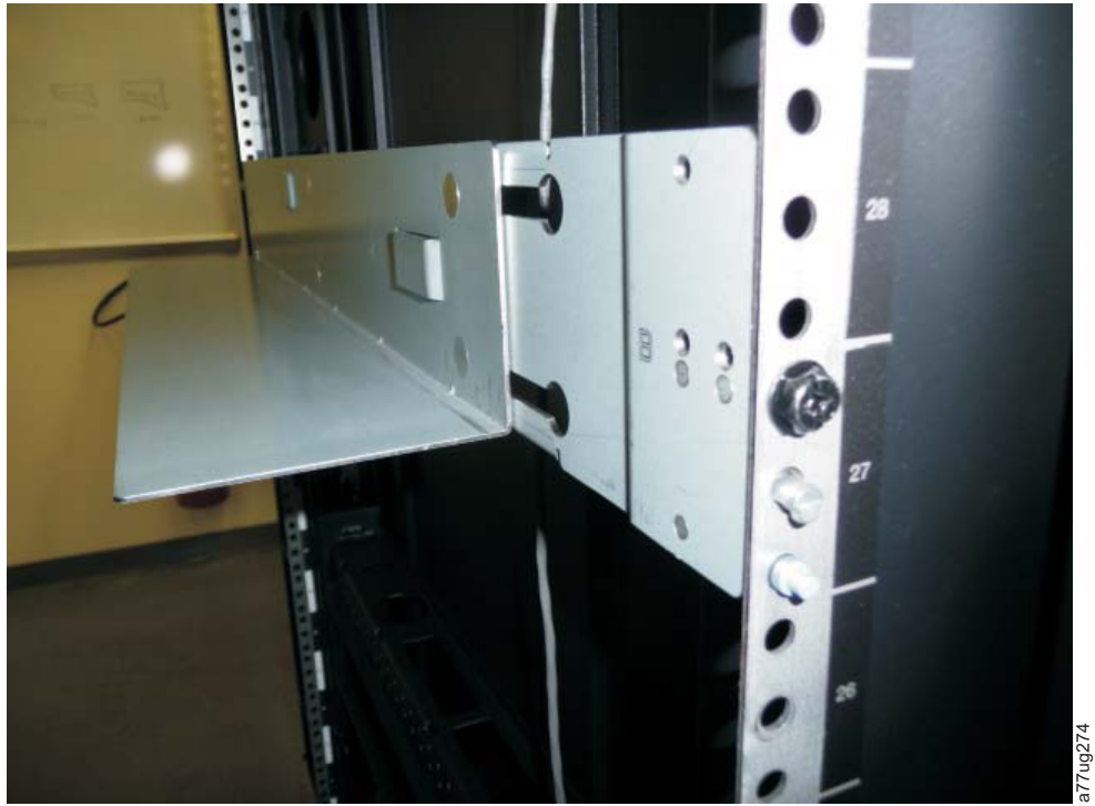
Figure 4-7. Alternate rear view of a rack showing the narrow part of the rail
