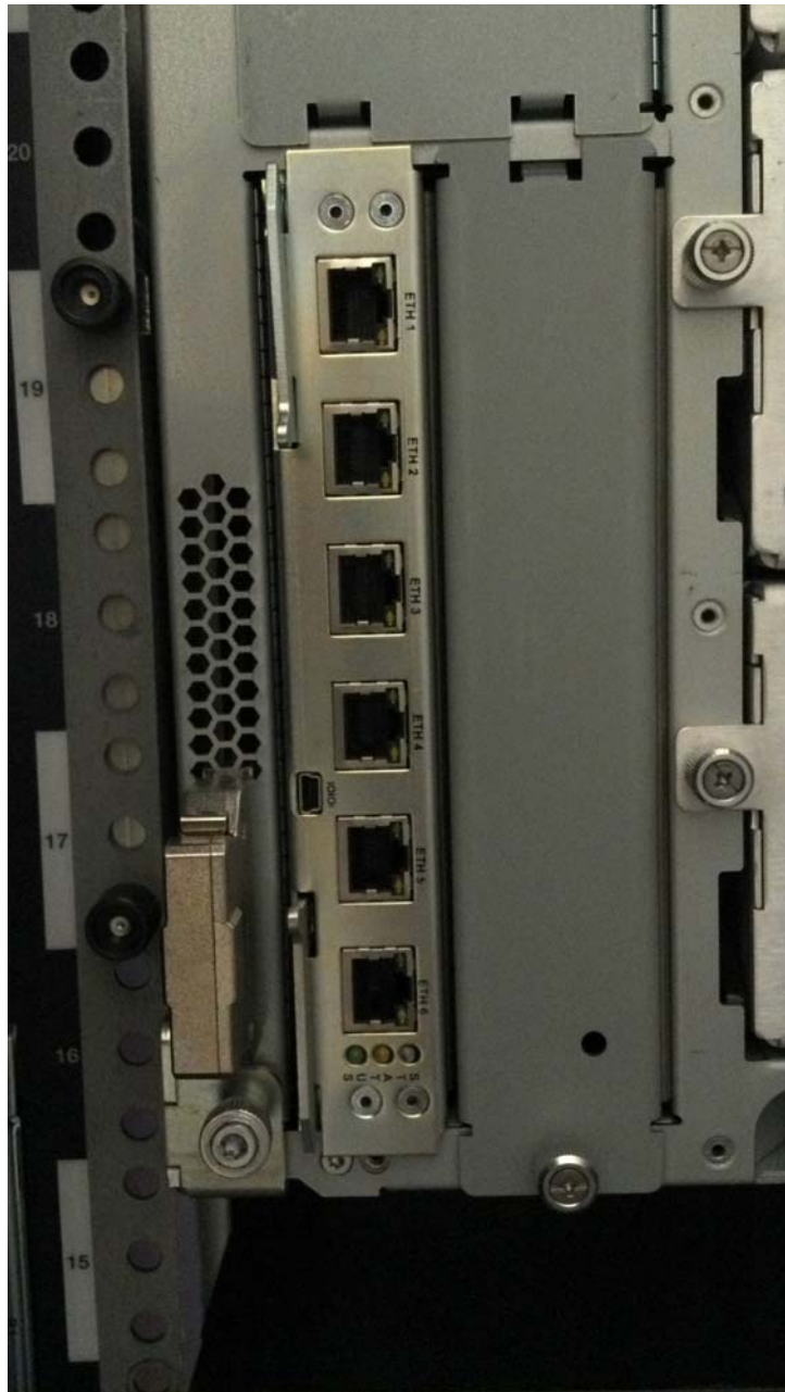
Figure 12-33. Ethernet cables removed
